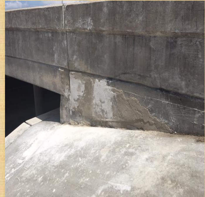
5 hr.'s Later Repair Completed
