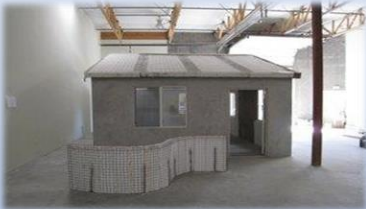
A prototype EkoRok Quik-Build structure using wire-mesh SIP panels, constructed by four people in three days.
