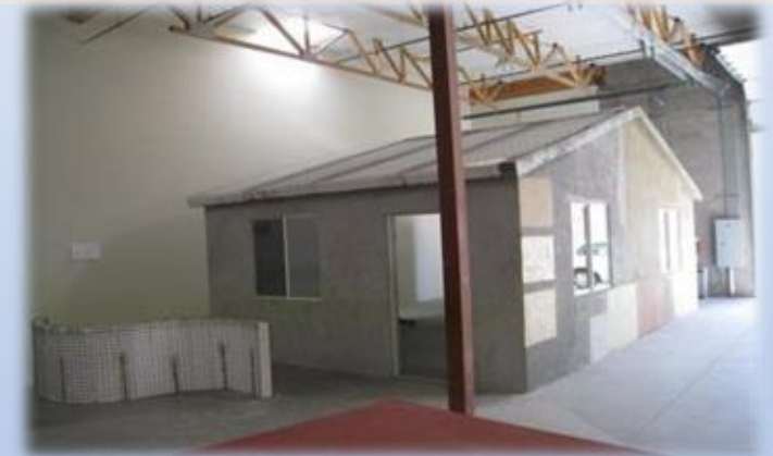
A prototype EkoRok Quik-Build structure using wire-mesh SIP panels, constructed by four people in three days.
