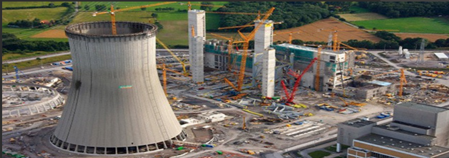
Traditional Portland concrete construction of a nuclear energy plant
