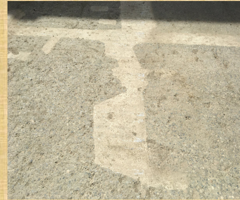
Nine-years after EkoRok repair, no spalling, no cracking
