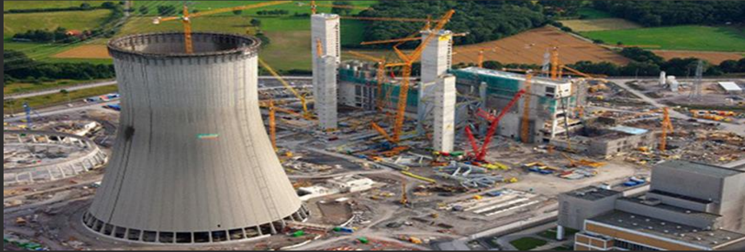
Traditional Portland concrete construction of a nuclear energy plant
