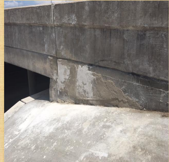
5 hr.'s Later Repair Completed
